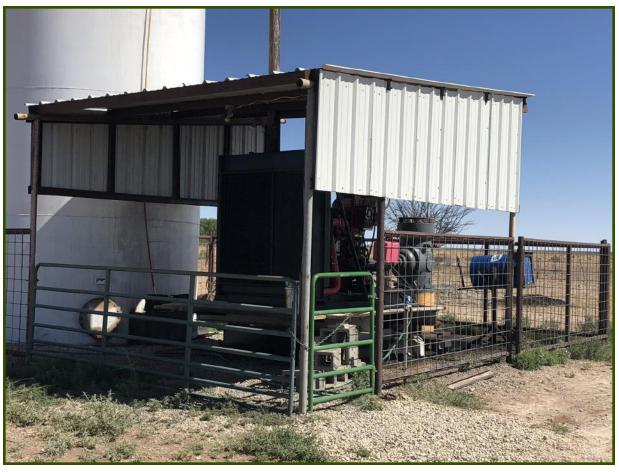
The well at the Williams Farm currently is on a diesel motor. This well waters 4 pivots at the same time if needed. This well is rated at 3300 GPM. In the near future, electricity will take the place of this motor.
