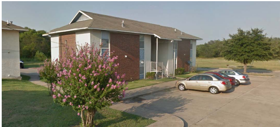
Undesirable - Inadequate Front Facade and Roof Articulation
