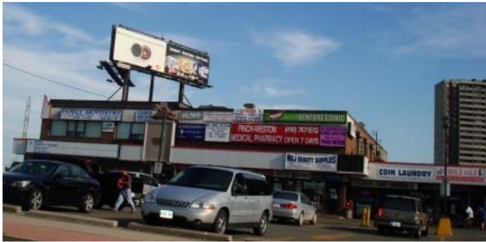
Undesirable design attributes – projecting flat upper façade with proliferation of unattractive signage and very obtrusive roof billboard
