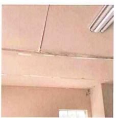
Signs of moisture was identified at ceiling areas. The inspection couldn't determine the cause or condition of underlying materials.
