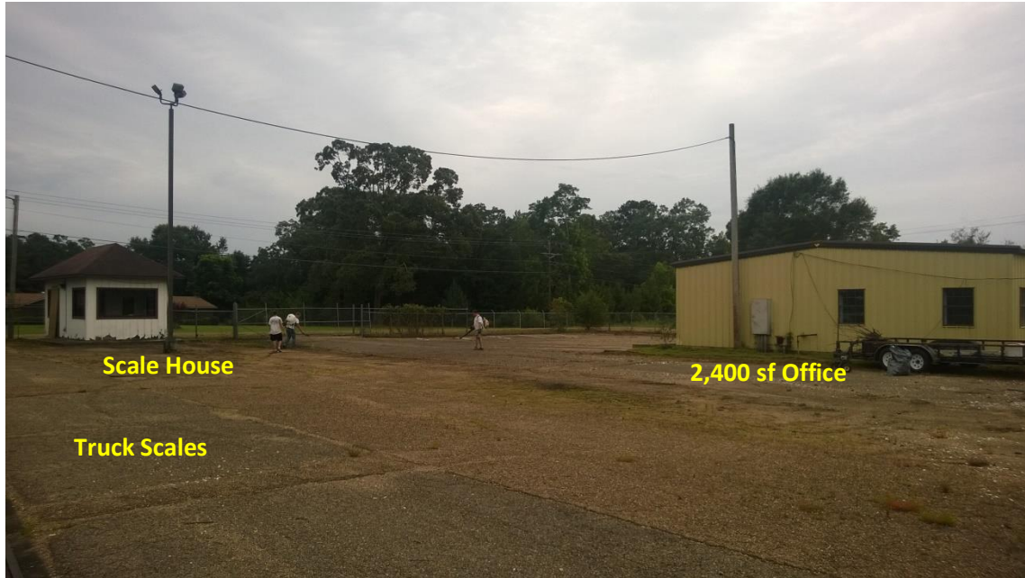
4) Scale House and front parking lot
