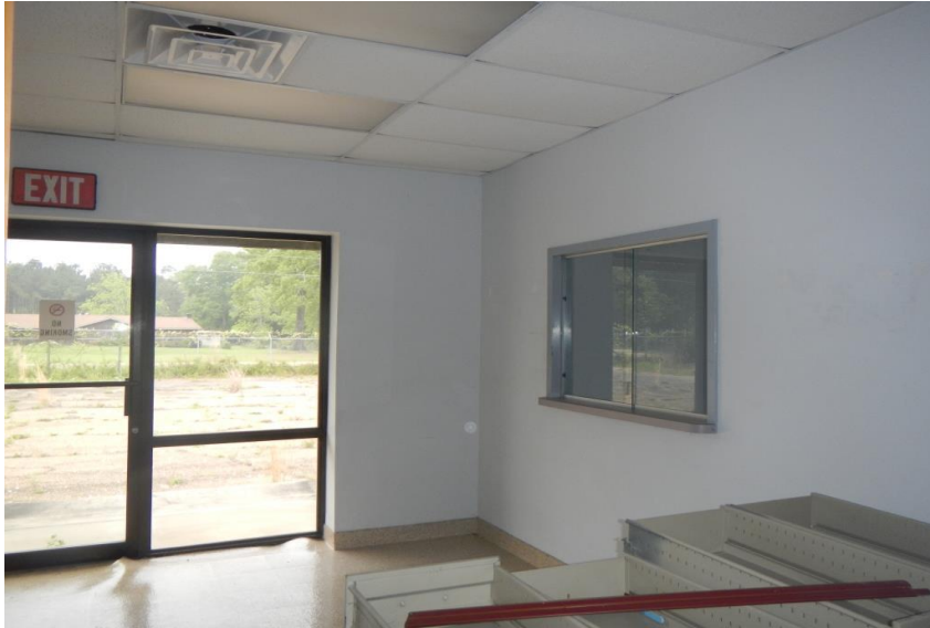
1) Front entrance with reception area
