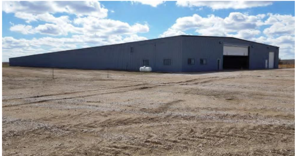
600' x 100' machine shed at the headquarters
